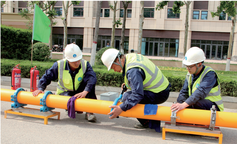
抢修燃气管道演练
