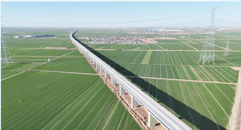
雄商高铁阳谷段架梁
